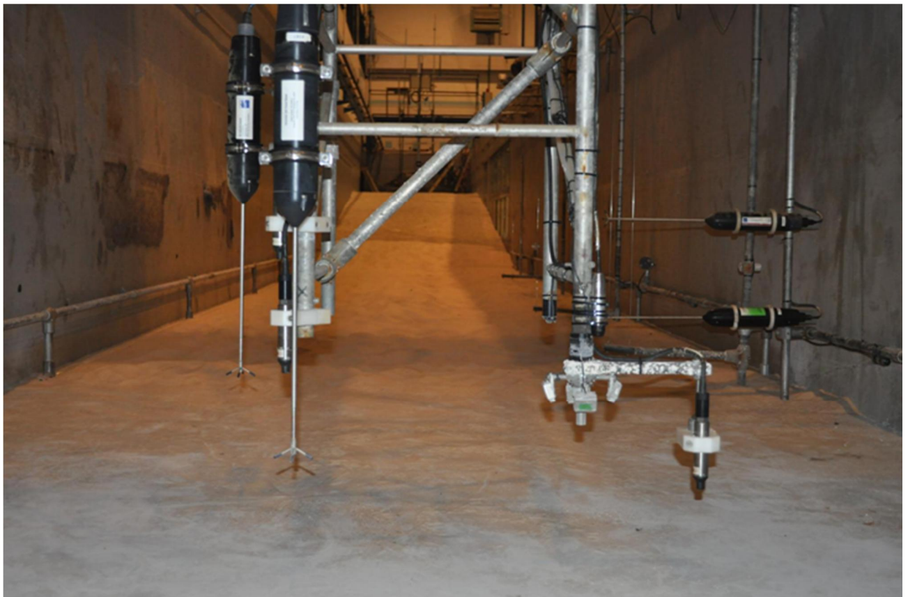
Figure 4: Image of the mobile measuring frame instrumentation.
